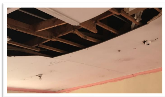
Image 2: Collapsing Roof: Gede Primary
