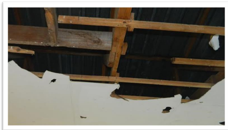
Image 3: Collapsing Roof: Rivoningo Primary
