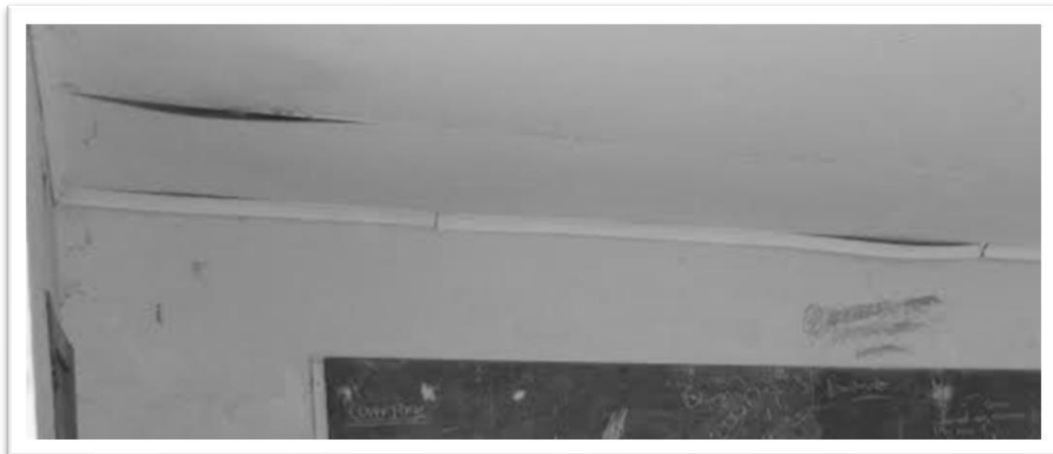
Image 4: Collapsing Ceiling: Tlanga Primary
